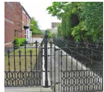
Railings and gates
